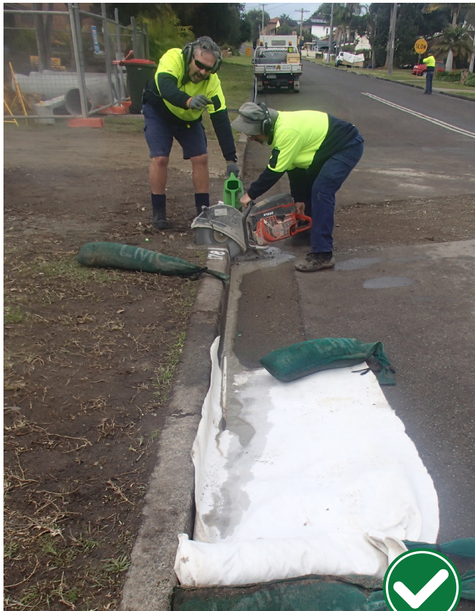
Agg bags and geofabric to catch sediments
