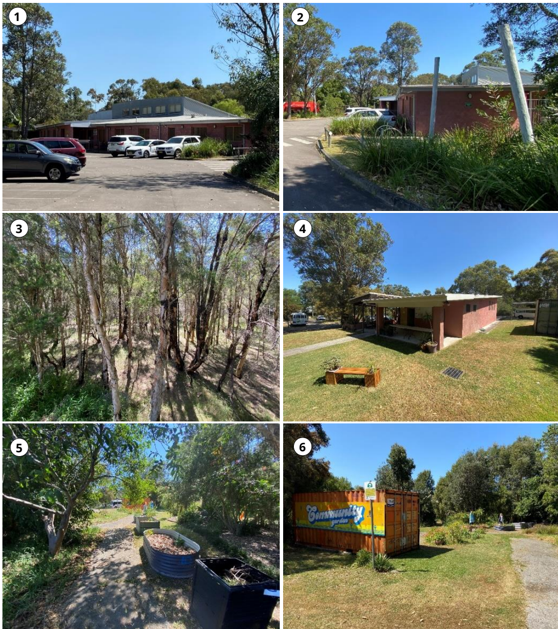
1 & 2 MULTI-PURPOSE CENTRE CARPARK AND BUILDING BEHIND
