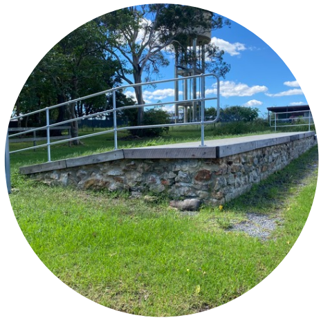
Livestock loading area
