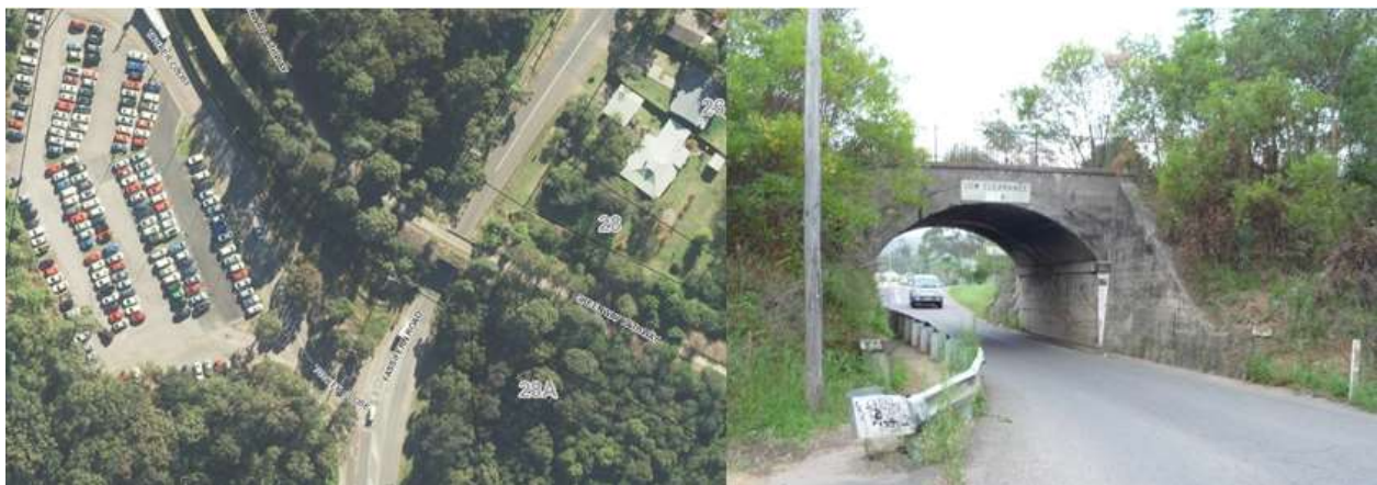
Figure 2.1: Fassifern Road rail underpass
