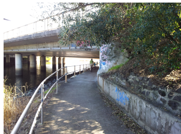
Photo left - shared pathway under highway at Kiama, NSW. A fence separates the creek
