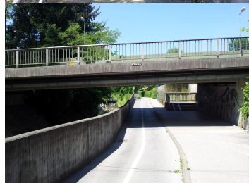
Photo left - shows a cycleway in both directions and pathway under a road. A concrete barrier separates the creek One of the above treatments may be suitable under Main Road at Glendale
