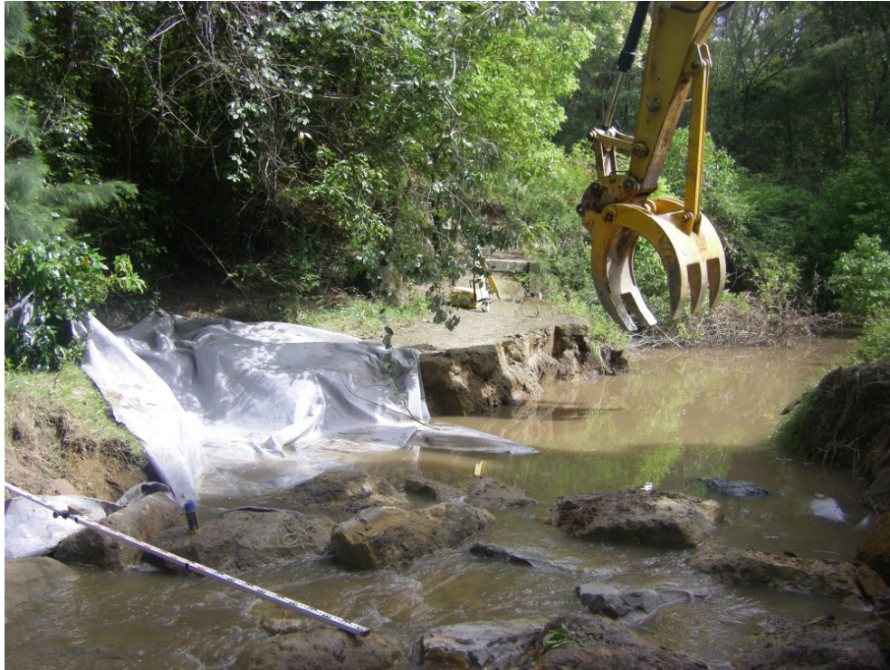
Figure 2.3 - Bed control structure being keyed into bank at Slaty Creek, Holmesville
