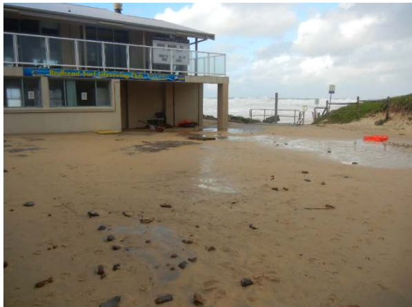
Plate 9.1a - Sand on the landward side of the Surf Club, due to waves overtopping the seawall.
