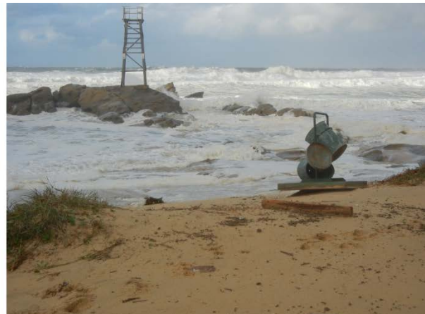
Plate 9.1b - Wave runoff at Redhead causing damage to bins on the beach.
