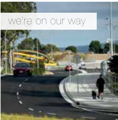
Stage 1 of the Lake Macquarie Transport Interchange was completed and opened to traffic in June
