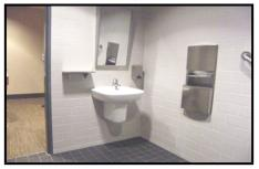
A good example of the installation of a washbasin and other fittings, including a shelf as required by Table F2.4 of the BCA, note that tilt mirrors are not a requirement of AS1428.1.
